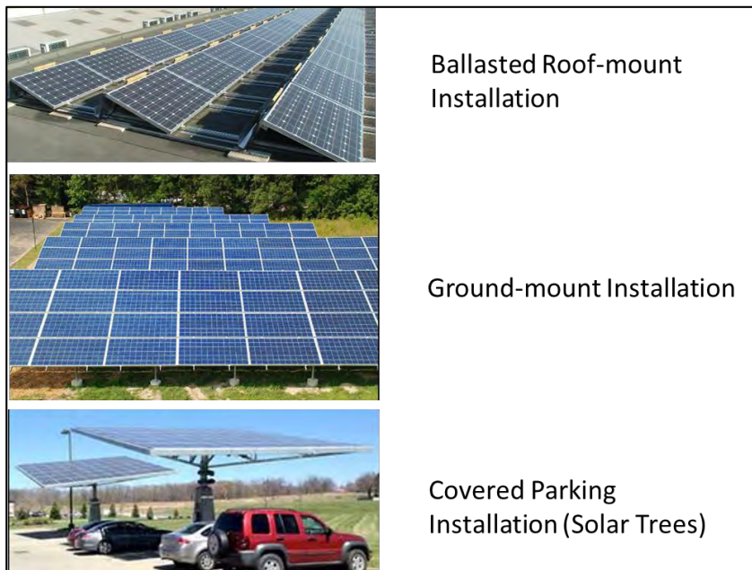
Figure 11 – PV Installation Options.
